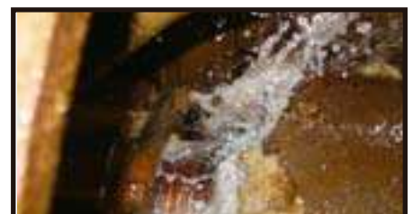
Gland packing 'slime out' consequences
